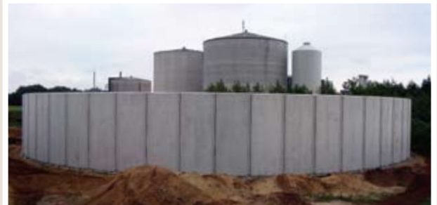
Tank installation period typically 1-2 days
